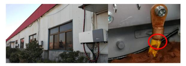
**Solution:** Create a gap at the bottom of the casing, allowing rain water to flow out Alternatively position the sleeve port outside the cable bay, prohibiting water from entering the inverter. In addition, the ground cable terminal connected to the AC side of the inverter must be treated with a heat shrink sleeve to prevent rainwater from entering the inverter through the ground cable sleeve.
