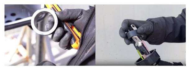
2 The diameter of the AC cable must meet the requirements, and the sheath processing is too long, the sealing ring pruning is too large, etc., will hinder the sealing cover's fit to the cable, resulting in poor air tightness.
