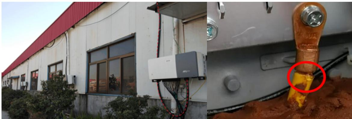
**Solution:** Create a gap at the bottom of the casing, allowing rain water to flow out Alternatively position the sleeve port outside the cable bay, prohibiting water from entering the inverter. In addition, the ground cable terminal connected to the AC side of the inverter must be treated with a heat shrink sleeve to prevent rainwater from entering the inverter through the ground cable sleeve.
