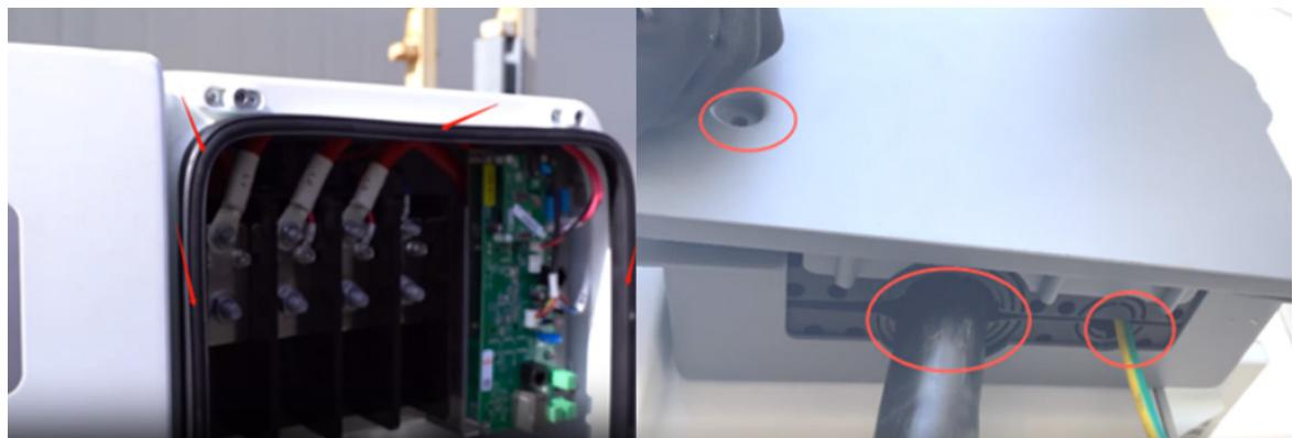
**Example:** External water enters the inverter through the pipe or cable. In some field installations, the communication line, AC line, ground cable and other cables have protective sleeves outside, one end of which extends to the inverter wiring bin, and the other end is often high and has an opening, so that rainwater can flow into the inverter through the pipe.
